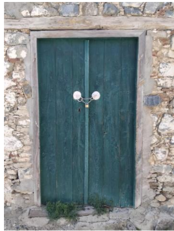
Door with double leaf timber planks
