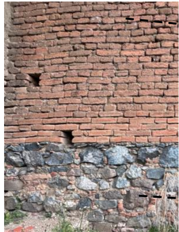
Wall build of large irregular igneous rocks with smaller stones and bricks
